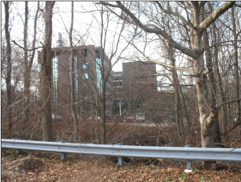
Photograph 8: View looking west toward 6-story Life Sciences Building from Nicolls Road adjacent to Project Parcel.
