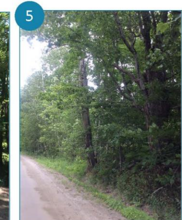
Tree roots damaged by ditching can lead to undermined slopes and tree decline. These trees in fair health and with low levels of mechanical damage from previous roadwork should be monitored yearly.
