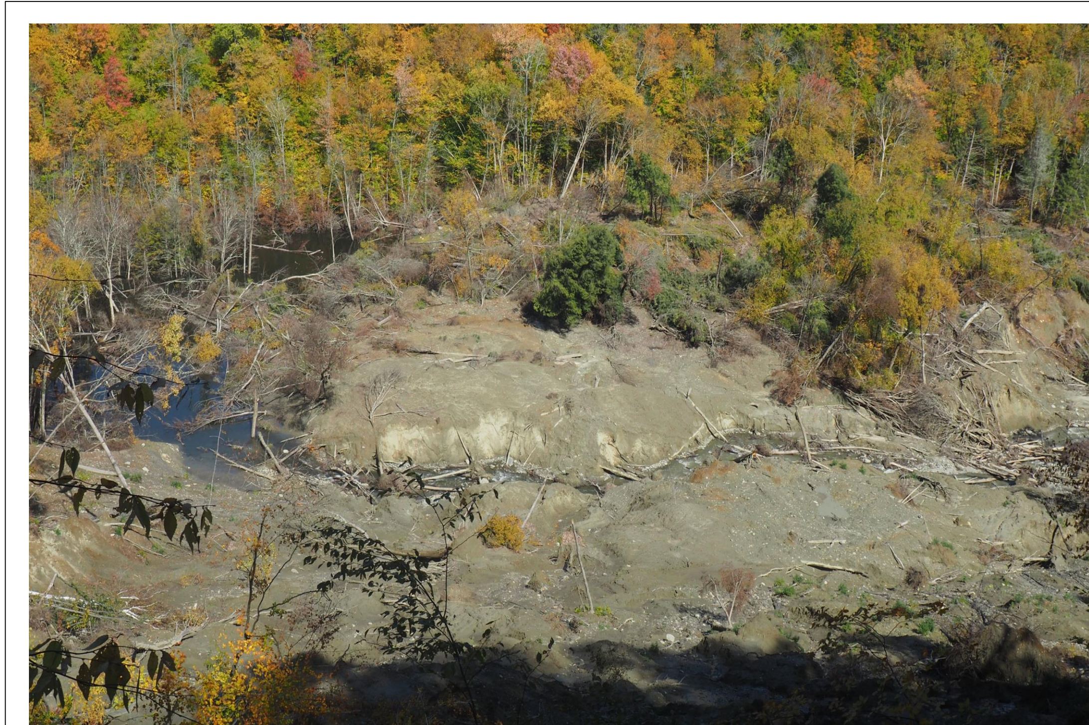
Fig. 4. October 8, 2019: View of the impoundment and the toe deposit. The pond extended upstream and encompassed approximately 1.8 acres.
