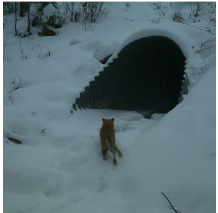
Figure 30 Example of structure that is ideal for wildlife crossing
